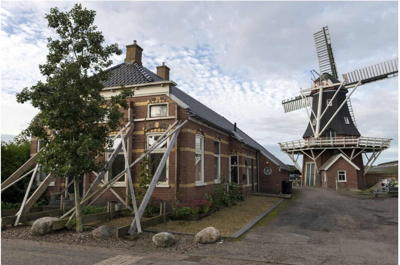
Hundreds of earthquakes have hit the Groningen region since the 1980s. Photographer: Imke Lass/Bloomberg
