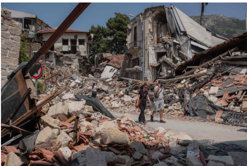
People on Sunday walked through debris caused by this year's devastating earthquake in Antakya. PHOTO: CAN EROK/AGENCE FRANCE-PRESSE/GETTY IMAGES
